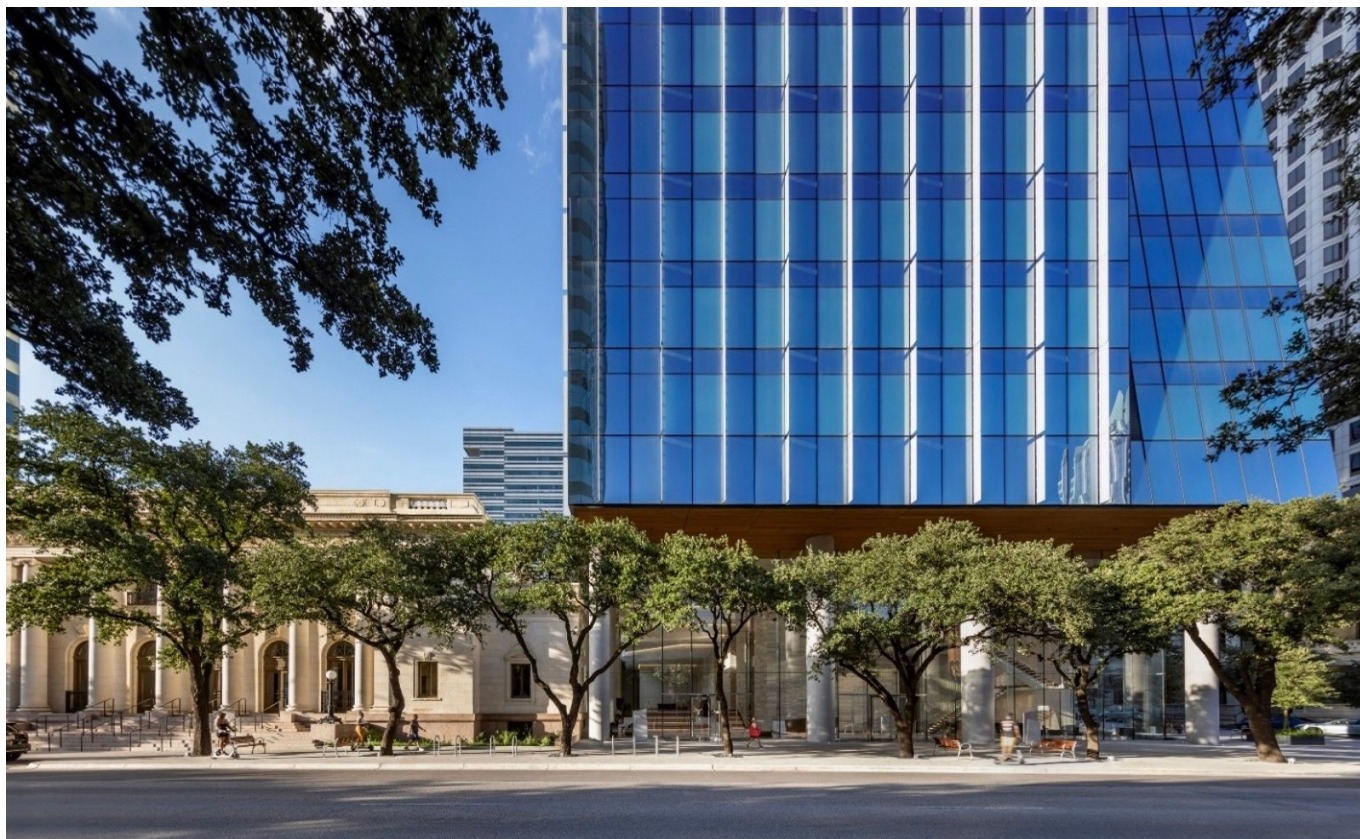
Claudia Taylor Johnson Hall is nestled next to Indeed Tower. Photo by Albert Vecerka/Esto.
